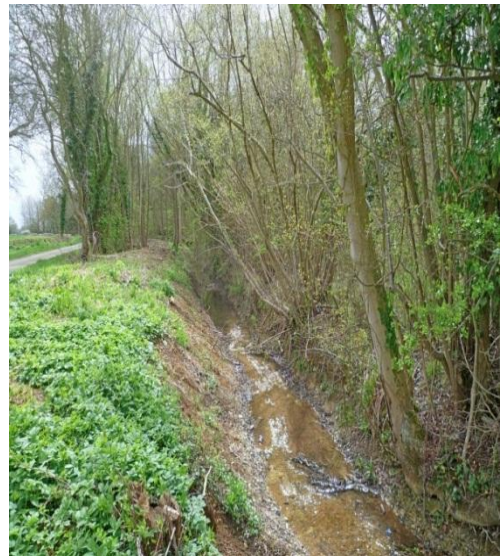
A newly slubbed out ditch
