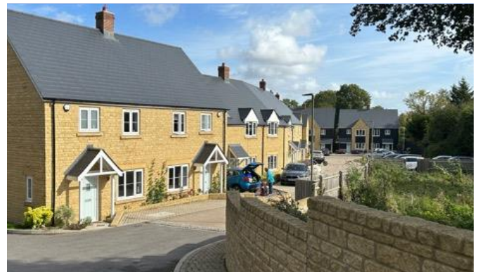
Canal Close – 14 stone-built properties with stone slate roofs, wooden casement windows and off-street parking. Note the varied roofscapes.
