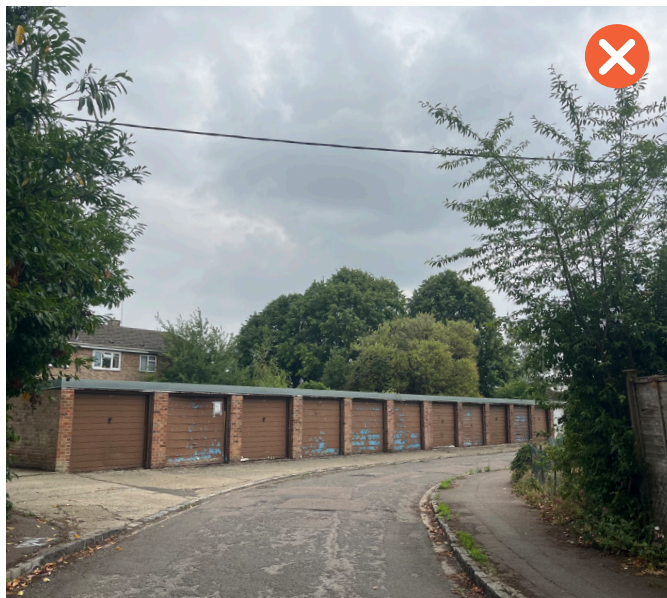
There are some very unattractive areas such as flat roofed garage blocks at Annersley Close which appear run down and face directly onto the street providing a dead frontage. These would be better sited and designed with more character sensitive development today as at Duchy Fields.
