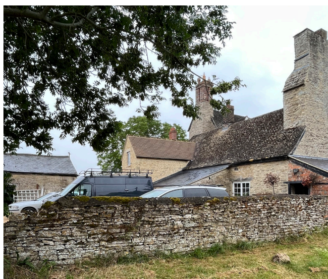
Views front and rear of the farmhouse
