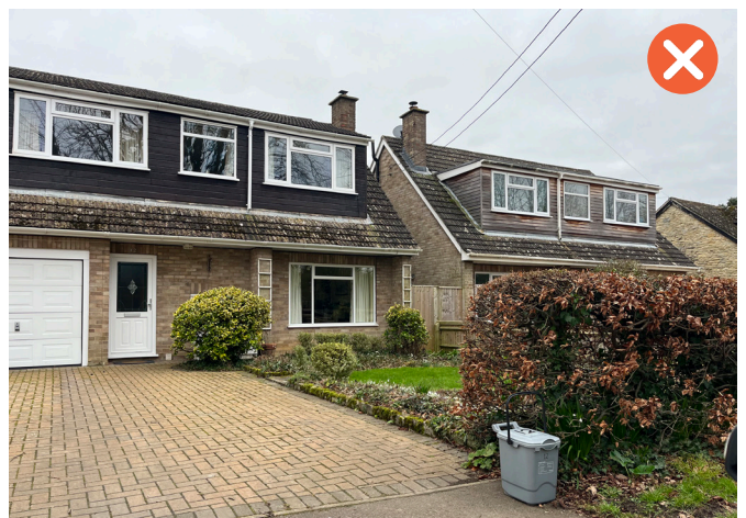
Chalet bungalows - Out of keeping with more traditional village character
