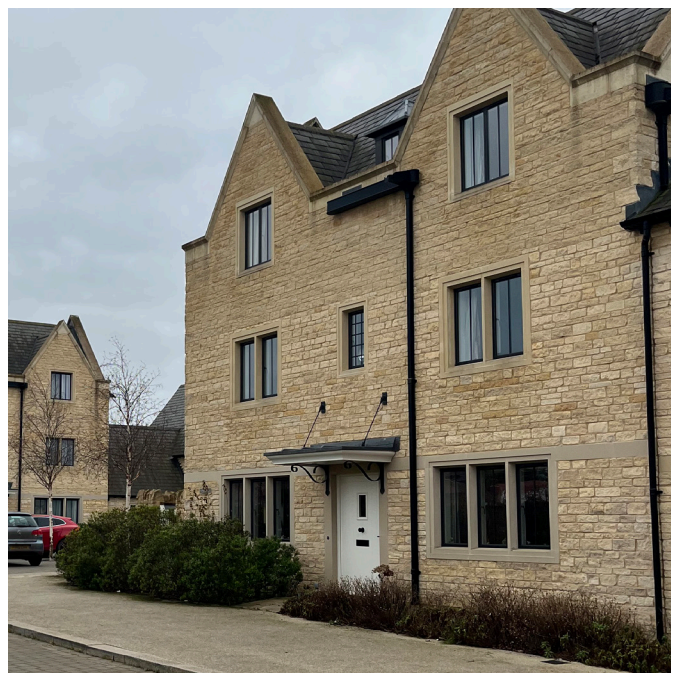
Application of coursed local limestone walling of random course heights and stone widths at Duchy
