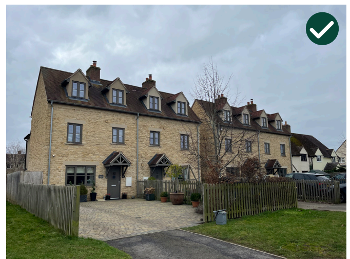
New terraced housing at Duchy Fields
