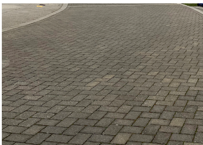
Block paving (not tarmac) with speed ramps with conservation kerbs. Tight radii to reduce speed. High stone boundary wall at corner reduces visibility and also helps to slow down traffic.
