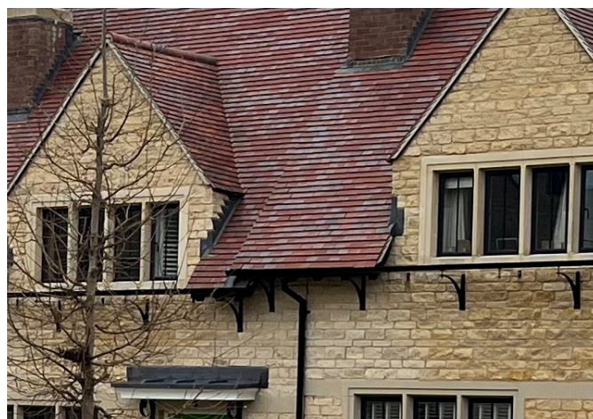
Generous eaves overhangs on brackets which add interest. Flush eaves detailing should be avoided. Chimneys add interest to the roofscape
