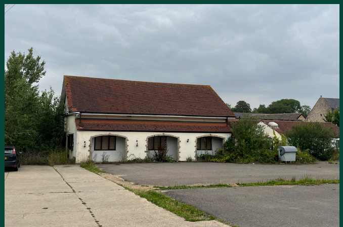
Former Oxfordshire Inn, now closed
