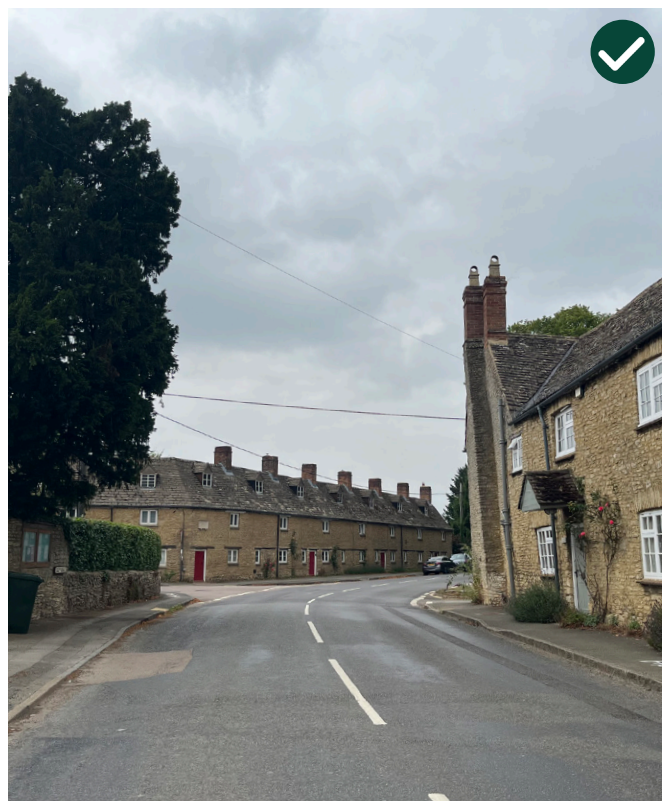
Cottages at Islip Road with The Row shown in the distance
