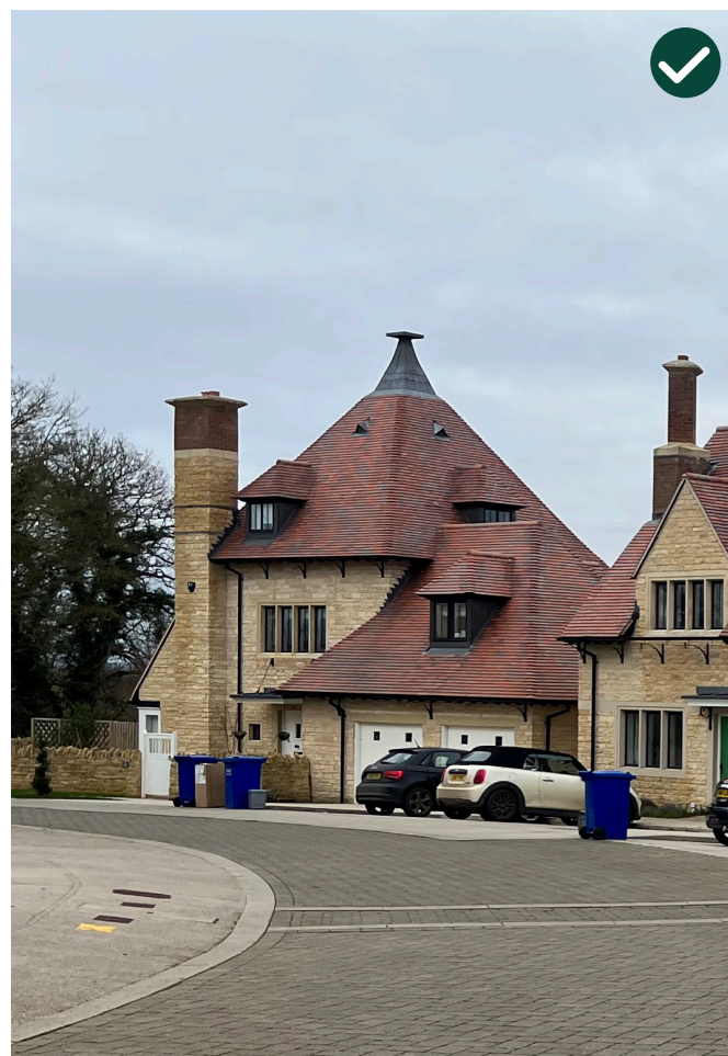
Lead clad hipped roofed dormers are characteristic of larger feature properties in dominant positions as above.
