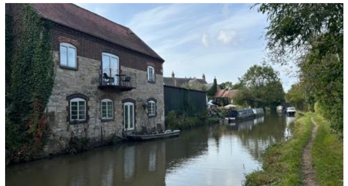
Old Stop House viewed from north bank of canal adjoins commercial uses in an important canalside location.
