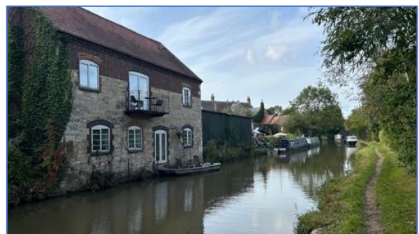
Figure 58 - the old Stop House, viewed from the north bank of the canal, looking south west
