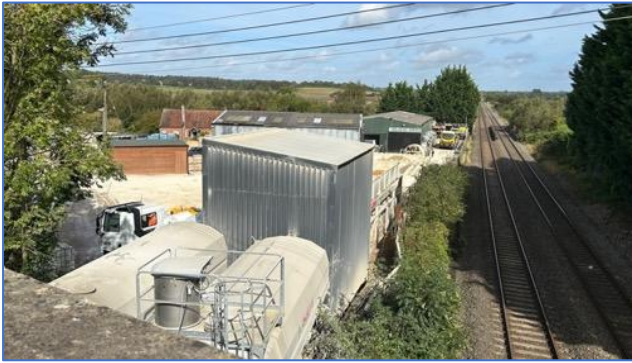
Figure 65 - the cement works
