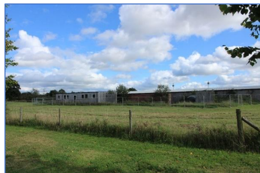
Figure 78 - abandoned golf driving range
