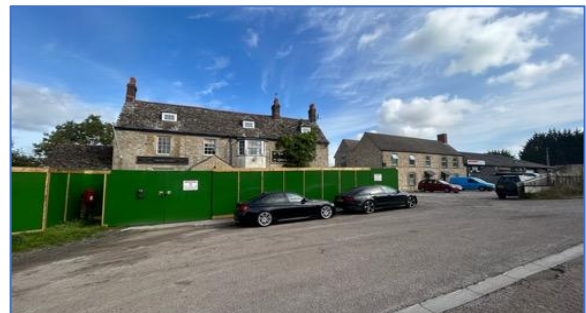
Figure 56 - the currently boarded up Rock of Gibraltar pub, viewed from Station Road
